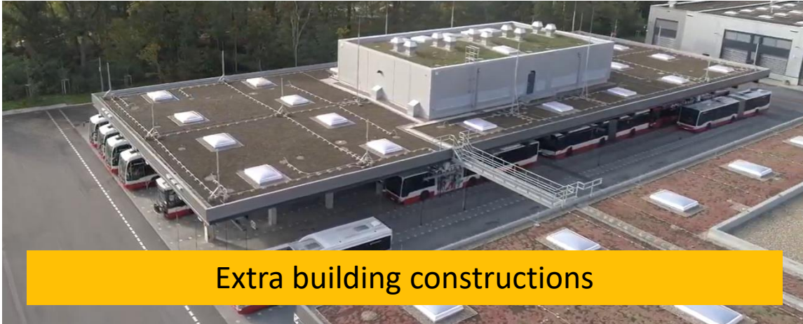
Depots for electric busses
