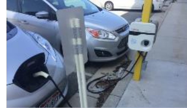
No cable damage
