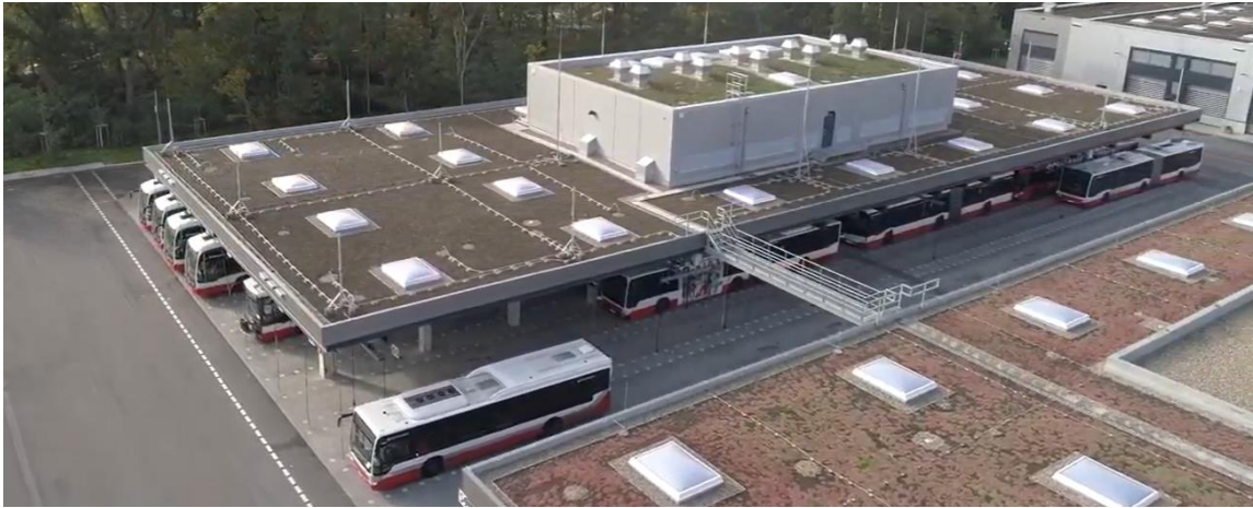
Depots for electric busses
